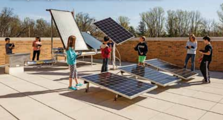
The rooftop Solar Lab at the Discovery Elementary School allows students to interact with a variety of renewable energy systems to engage in experiential learning and support the curriculum. Photo by Lincoln Barbour.
